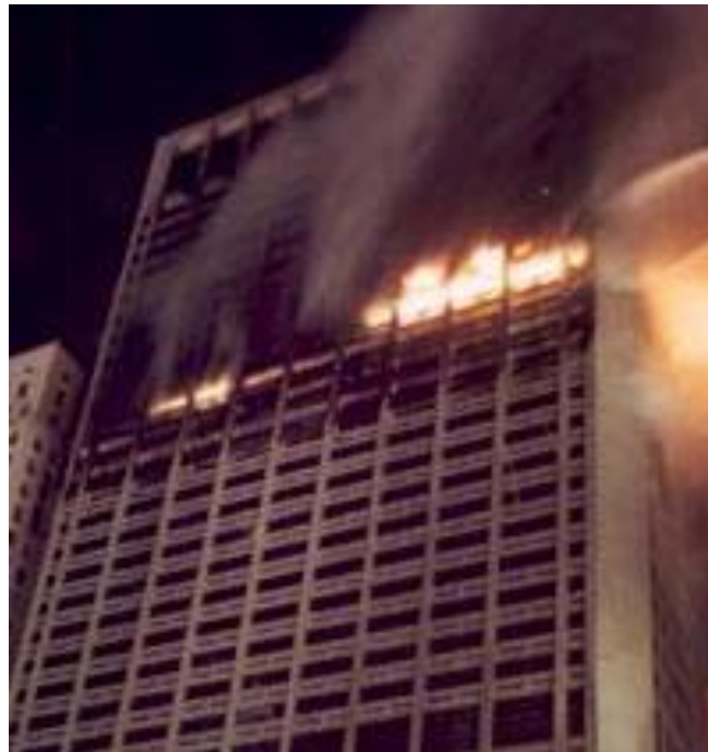
Figure 40. On 23 rd February 1991, One Meridian Plaza, a 38-storey skyscraper in Philadelphia, was subject to raging fires for 18 hours, causing
