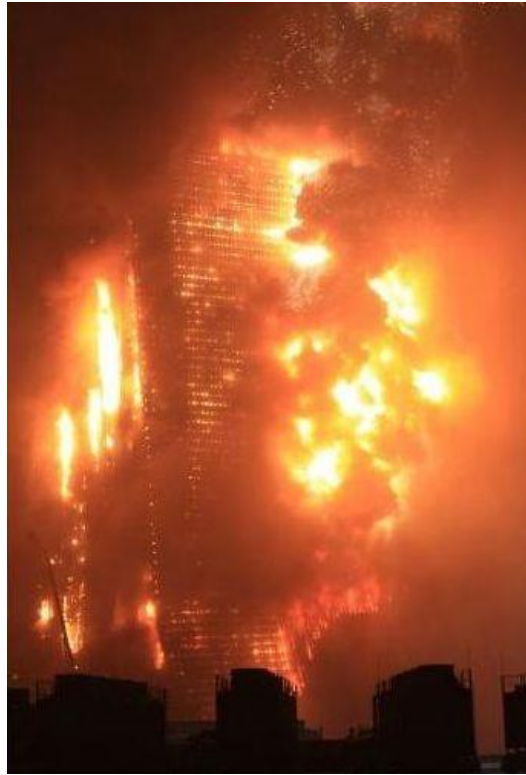
Figure 43. On 9 th February 2009, the Hotel Mandarin Oriental 520-foot-tall skyscraper in Beijing, was engulfed by fire for at least three hours, no large portion of the structure collapsed
