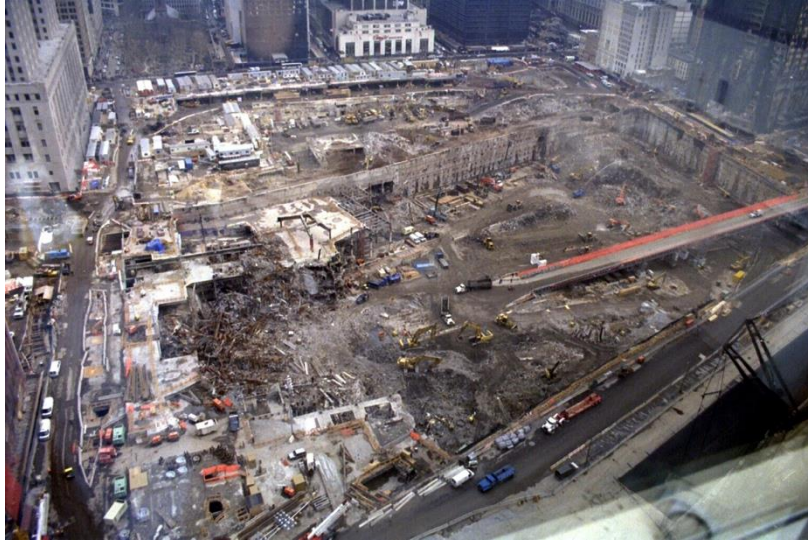
Figure 67. Wood's Figure 15: The nearly cleaned-out bathtub. (March 15, 2002) http://www.nytimes.com/2002/05/07/opinion/_07TUE1.html?ex=1159329600&en=40a1d614eadcfc0&ei=5070
