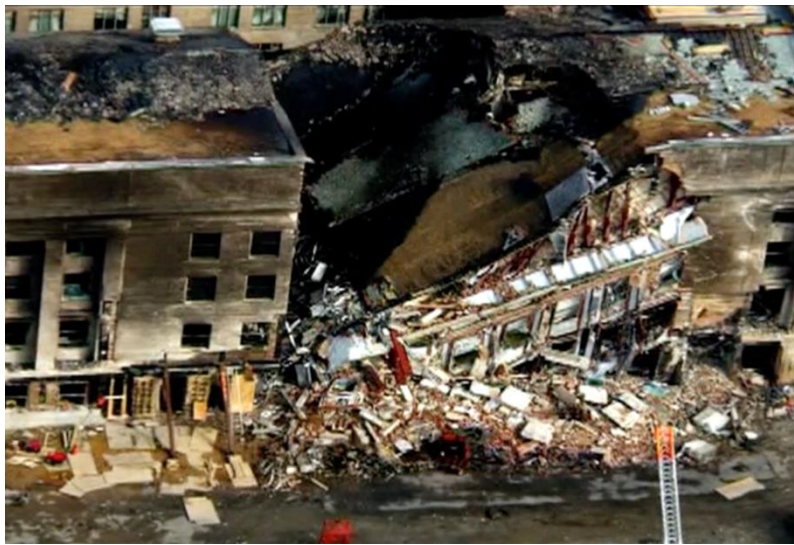
Figure 13. Image of the Pentagon taken shortly after the impact of the object and the collapse of the façade. There are no visible parts of a jet airliner
