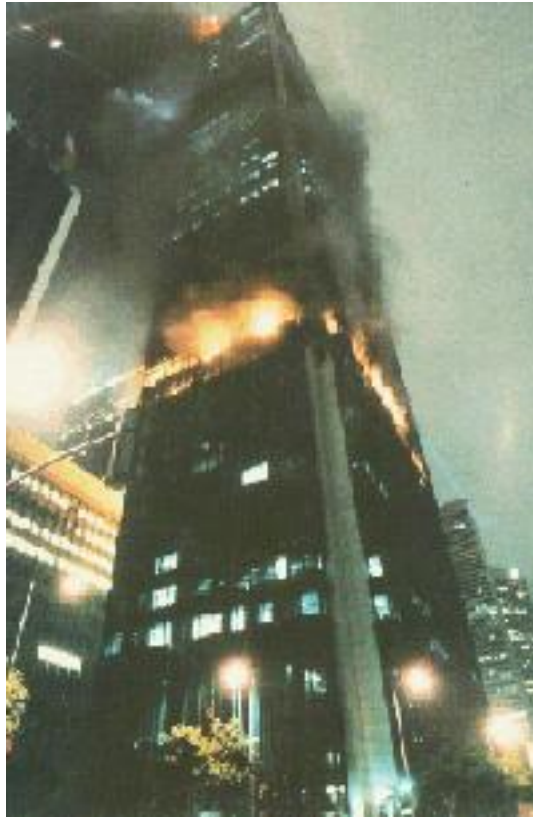
Figure 41. On 4 th May 1988, the First Interstate Bank, a 62-story skyscraper in Los Angeles caught fire for three and a half hours. In spite of the total burnout of four and a half floors, there was no damage to the main structural members and only minor damage to one secondary beam and a small number of floor pans.
