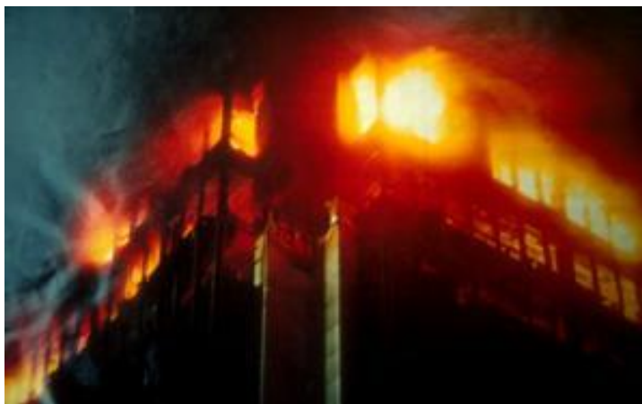
Figure 42. On 5 th August 1970, 1 New York Plaza, a 50-story office tower less than a mile from the World Trade Centre complex, burned for more than
