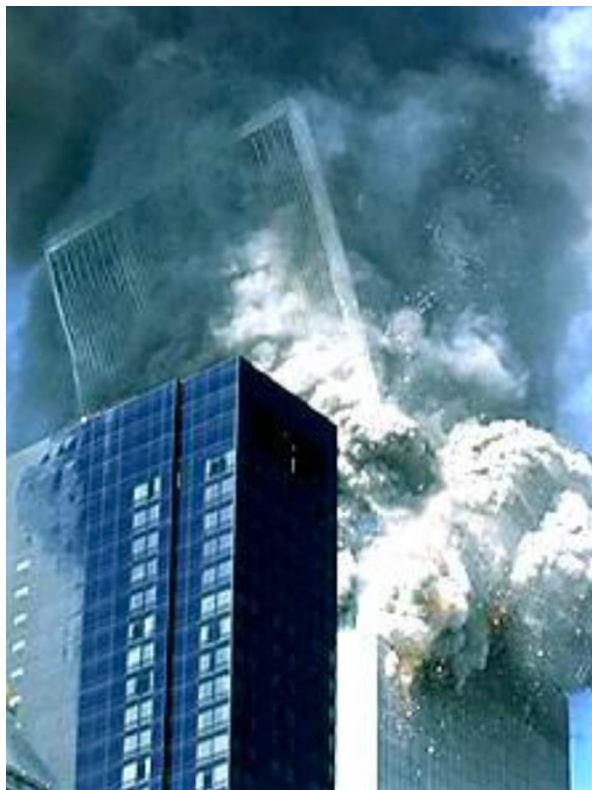
Figure 45. An image of the beginning of the collapse of WTC2, showing about thirty storeys of the building toppling over
