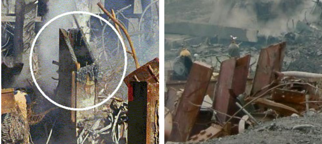
Figure 46. Details of two images from Jones's research, page 32, showing remaining steel columns cut at an angle of 45 degrees, a feature of controlled demolition using thermite/thermate
